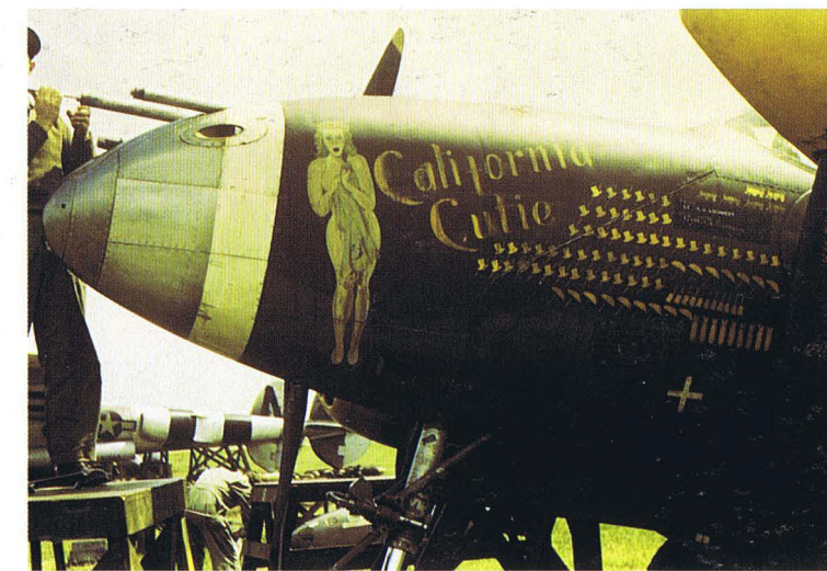
T/Sgt. Thomas Dickerson cleans the guns on California Cutie , a 55th Squadron, 20th Fighter Group P-38J, code KI-S, flown by 1st Lt. Richard O. Loehnert. The white band and polished nose were meant to confuse enemy pilots on whether the Lightning was a Droop Snoot or not. The mission symbols stood for many different things: locomotives for those claimed in strafing, bombs for fighter-bombing missions, brooms for fighter sweeps, umbrellas for top cover, top hats and canes for bomber escort. John W. Phegley
