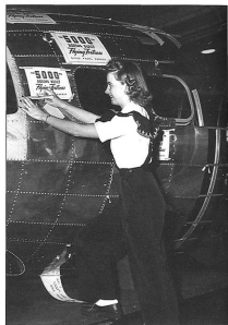
ABOVE As the nose of 43-37716 comes out of the assembly jig, a worker affixes appropriate posters to the unit. Note the bare metal finish, although the cheek gun assembly (extreme left) has been sprayed in zinc chromate
