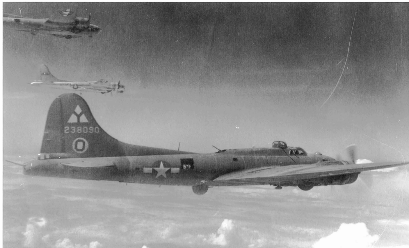
Above and below are unnamed B-17s of the 97th Bomb Grp., Fifteenth Air Force. Note the unique, late model, radar dome in place of the belly turret on #297731.
