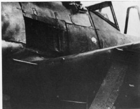
Fw 190A-8 showing MG 151, camera, and MK 108 at the wing front.
