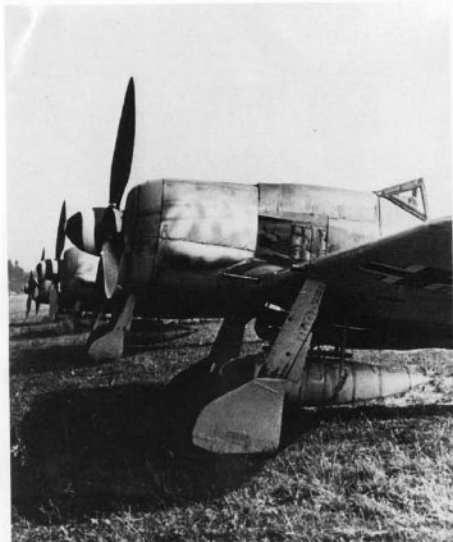
Fw 190A-8 of JG 300 with MK 108 armament. Note stenciling on the aircraft and on the auxiliary tank, "keine Bombe."
